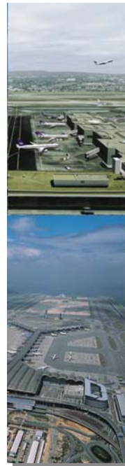
Charles de Gaulle Airport (France)
